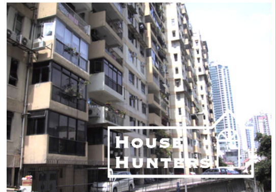
Merry Terrace, 4A-4P Seymour Road, Mid-Levels
